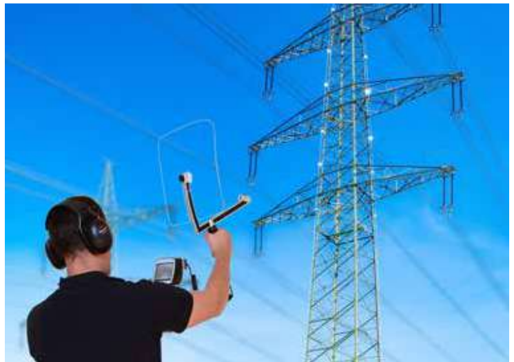
Checking high voltage overhead lines for corona discharge
